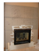
Wire Mesh applied over drywall.
