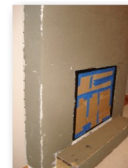
Scratch-coat of mortar applied.
