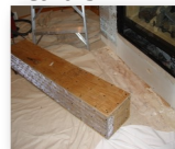
Building a new hearth out of plywood, followed by wire mesh, anchoring to floor, scratchcoat, then stone.
